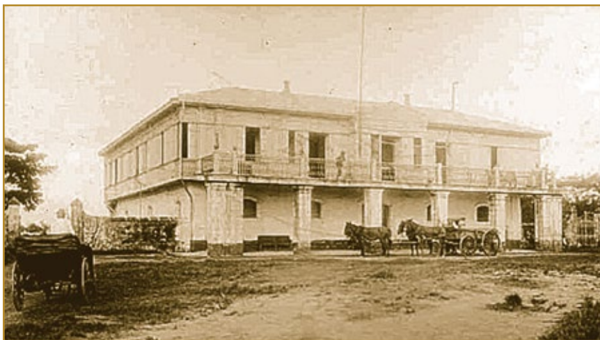
The El Deposito is the centerpiece of Manila's waterworks in 1880. Water was pumped from the Marikina river to San Juan and flowed by gravity to different points in Manila.
